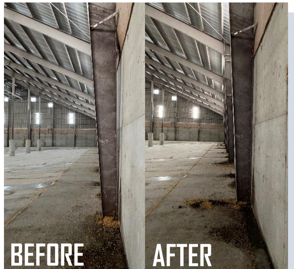
Grain bin interior wall before & after lift
