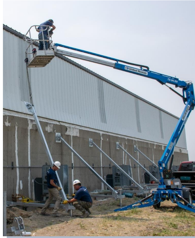
Installation of buttresses
