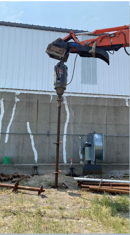
Installation of Helical Piers
