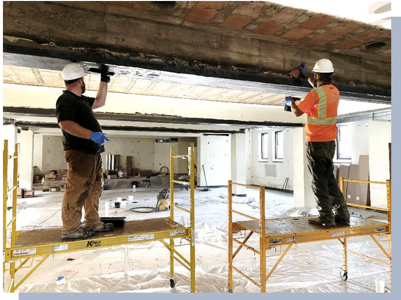
Left: Surface Prep Above: Epoxy Application
