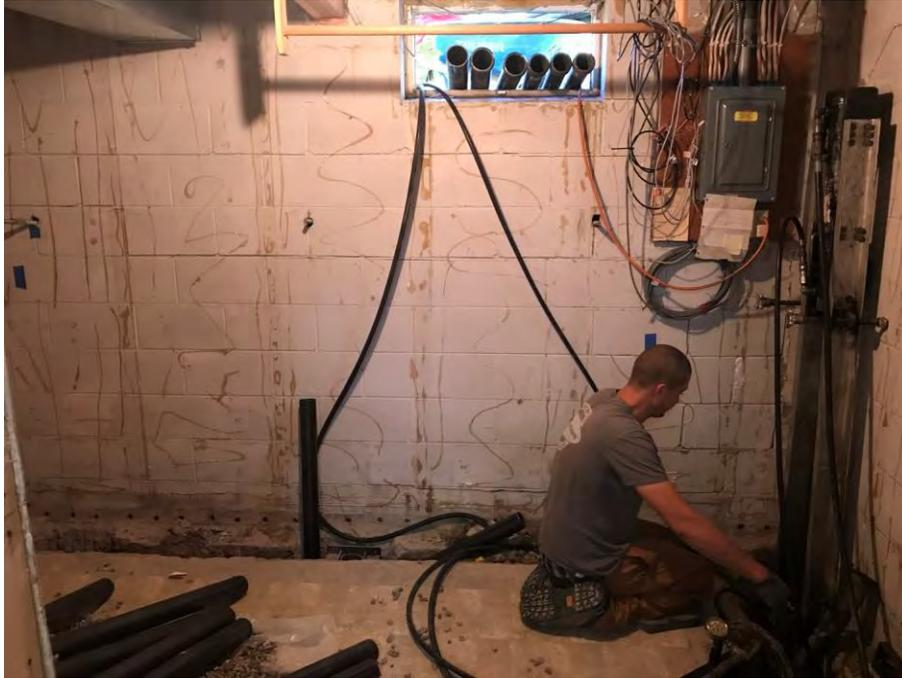
Wall anchors were installed on the west wall to prevent further bowing, and give the ability to straighten the wall. SafeBase push piers with SaberTooth bracket assemblies were used, allowing for a low profile installation, and the advantage of not having to shim the bracket in the waterproofing trench.
