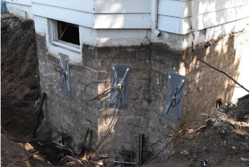
During installation portions of the foundation began moving outward. Temporary tie backs to the interior were installed using large wall anchor plates, cables and turn buckles attached to steel plates bolted to the slab. The tension was adjusted so that the walls would stay together and not displace laterally during the lift.
