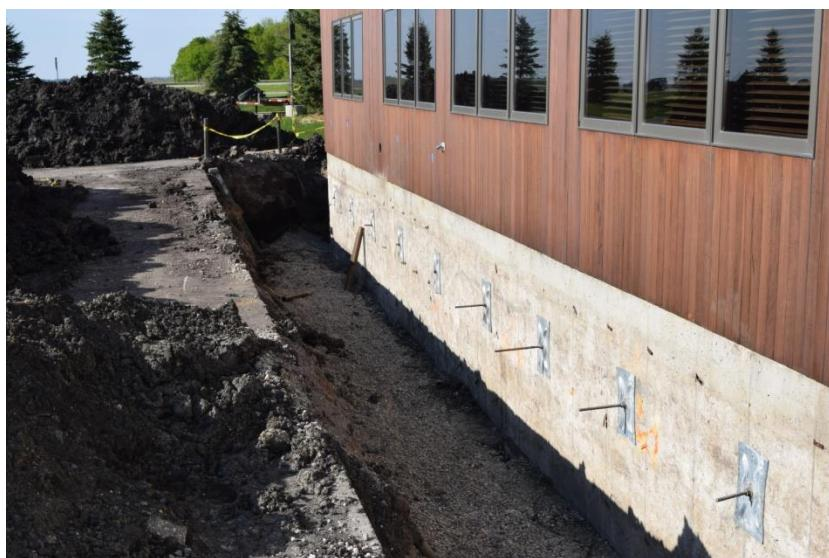
Along the western wall of building three, a total of 15 SafeBase™ Wall Anchors were installed. Before the lift of that portion of the building, cables with turnbuckles were added along the north and south foundation walls. The anchors and turnbuckles were then used to pull the foundation wall back to plumb while the lift cylinders were raising the wall. With the wall back in place, the brackets were tightened and the cables removed.
