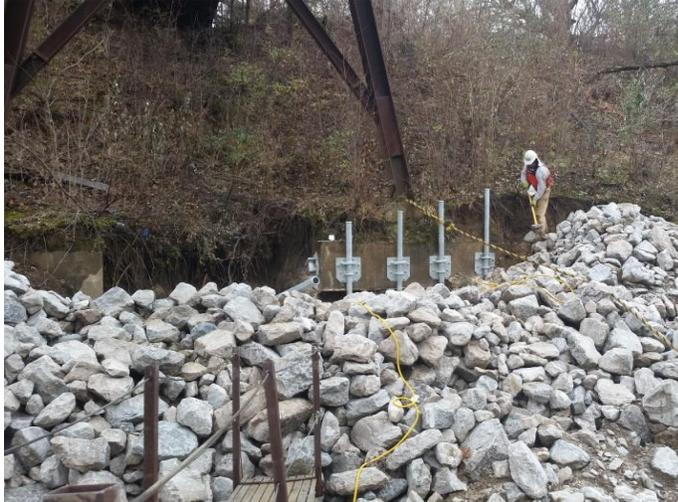
A site visit revealed that one of the four footings had an undermining issue. To prevent any further soil loss rip rap would be placed on the failing slope. In addition it was decided that 4 push piers be installed on the face of the footing. Another on the narrow side would be installed with a 30 degree batter. Although this won't do anything for load it will prevent any future downhill movement.
