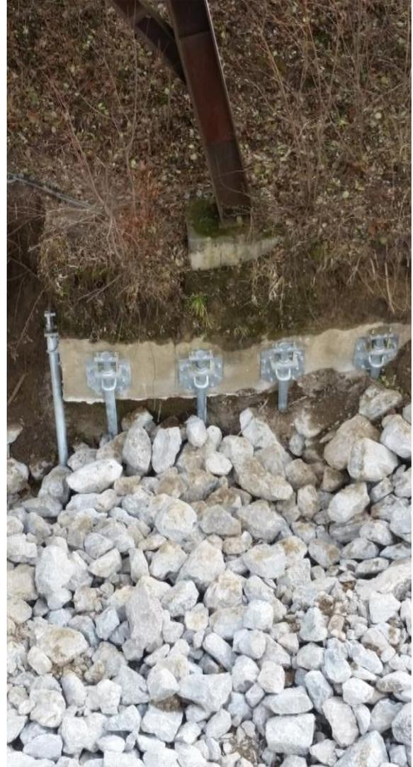
Installation went very smoothly with the piers reaching a 30 to 40 foot depth and pressures slightly above 4,000 psi or 38,000 lbs of force. Lift cylinders were then attached and movement was observed at slightly less than 9,000 lbs of force. The safety factor was greater than 4.
