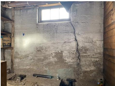
A plan was made to support the foundation with SafeBase™ 2.875" OD Standard Duty Push Piers with SafeBase™ SaberTooth™ Bracket Assemblies. A total of 22 Push Piers were installed
