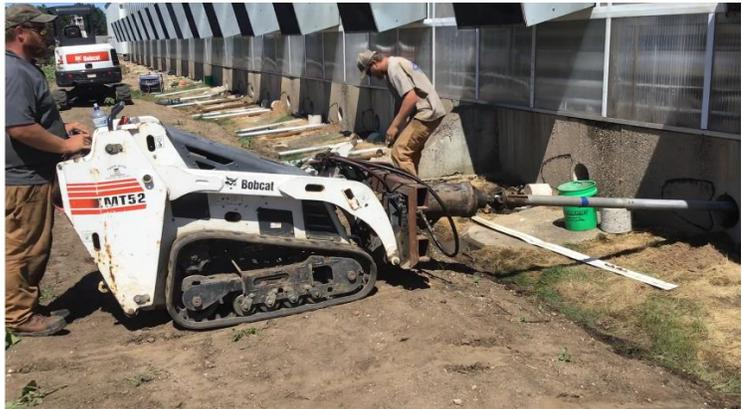
A total of 62 Helical Tiebacks were installed. First, 10" holes were core drilled into the face of the wall, then helicals were screwed in through the wall to the specified torque. After the helicals were installed a tieback adapter was attached to the pier shaft with threaded rod extending out beyond the wall. The hole in the wall was patched and plates were installed on the exterior.
