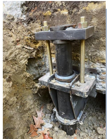
Installed SafeBase Push Pier
