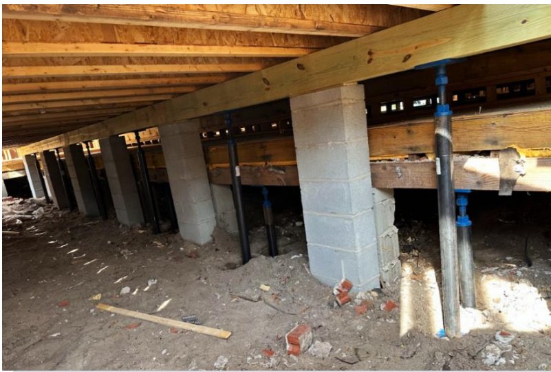
SafeBase Stabilizers on Existing Footings
