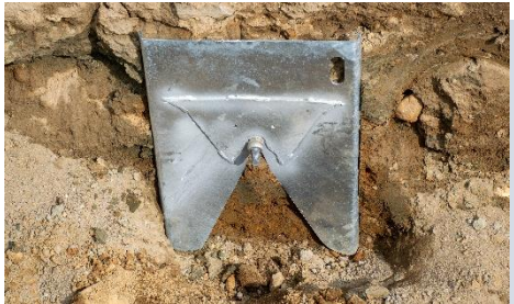
Top: Pulling back wall Bottom: Installed earth plate
