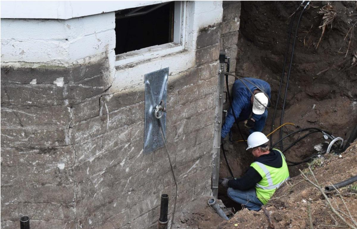
SafeBasements of Minnesota was contacted regarding concerns of cracks in a foundation wall during renovation of the home. It was found that the northwest corner of the home was down approximately 2.5". A plan was made to underpin the settling foundation using SafeBase™ 2.875" Standard Duty Push Piers. The piers needed to be installed and the foundation lifted before construction of a second story addition could be started.
