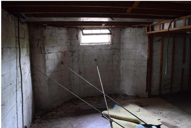
A full recovery of the 2.5" settlement was achieved during the lift, bringing the house back to level. After the lift all cracks in the foundation wall were tuck pointed and the holes made for the cables were patched on both the exterior and interior.
