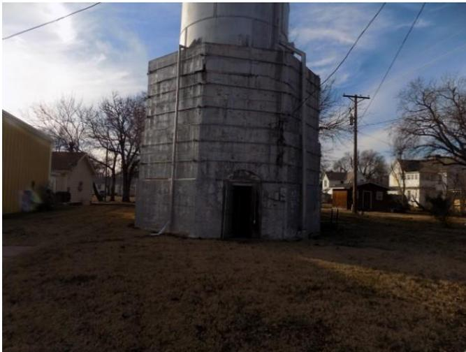
Lamunyon's solution was to use 24" bidirectional carbon fiber mesh to hold the base together. With a tensile strength that's nearly ten times more than steel and five times lighter. This is one repair that should hold up much longer. Two layers of the 24" carbon fiber bidirectional mesh were installed; one covering the surface oriented horizontally, and one covering the surface oriented vertically.
