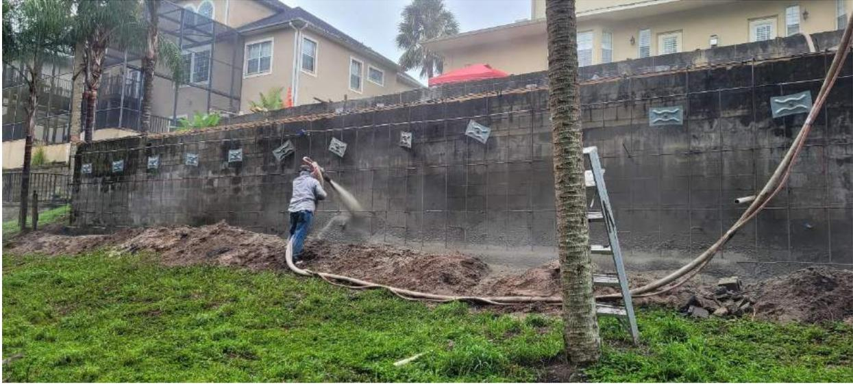
A grid of rebar was placed in front of the existing walls and behind the wall plates for the anchors and tiebacks. With the rebar in place shotcrete was applied to the wall.
