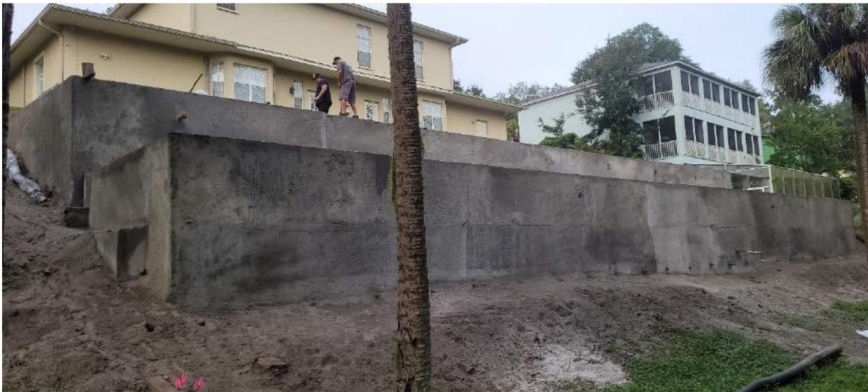
A beautiful new set of walls are now in place supported by 37 SafeBase Wall Anchors and 5 SafeBase Helical tiebacks. There will no longer be concerns of future displacement of the pair of retaining walls. The project completed September 2022.
