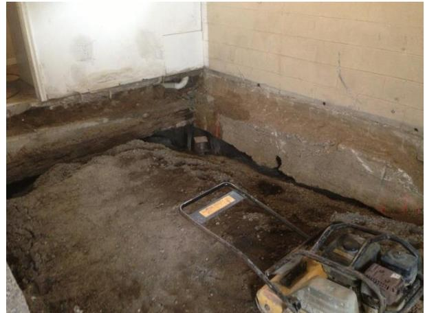
With the 9 SafeBase Standard Duty Helical piers supporting the new reinforced concrete 20"x20" grade beams and 7" slab the garage would be safe for parking multiple vehicles for the life of the home. The garage was able to be heated during construction allowing for the project to be completed in January of 2014.
