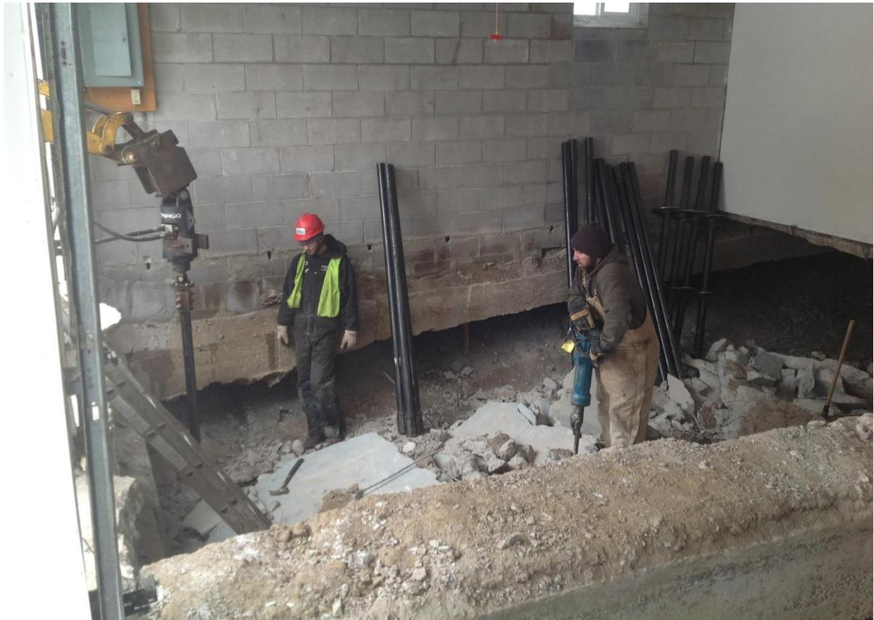
SafeBasements of Minnesota was contacted regarding concerns about a sagging garage floor. A plan was created by Wenzel Engineering which called for removal of the existing floor and replacement with a new floor supported by system of reinforced concrete grade beams and helical piers. The home was originally built on timber pilings in 1977 and over time the soil beneath the slab settled creating a 4-6 foot void beneath the floor.
