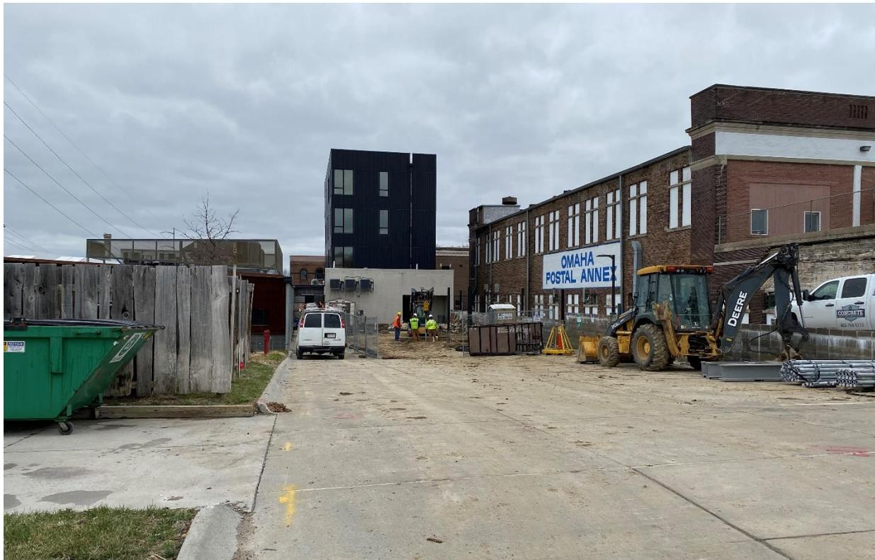
CLS was contacted regarding the installation of helical piers to support the grade beams for the addition to the Boxcar 10 building in Omaha, Nebraska. A total of 48 SafeBase Standard Duty Helical Piers with 10-12-14" flights were to be used to support the foundation. Each pier was to be installed to a torque of 7,086 ft-lbs to correlate to an ultimate bearing capacity of 60 kips.
