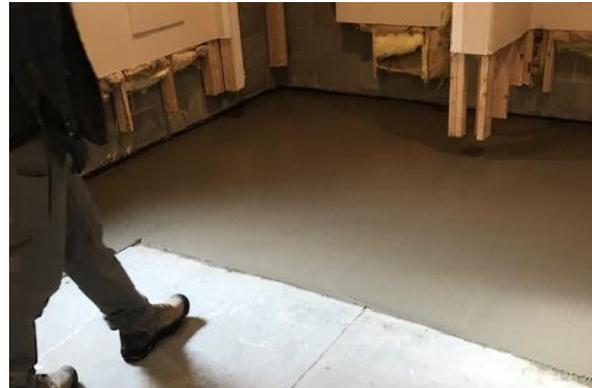
After the push piers and interior drain tile system were installed the concrete floor could be poured back into the basement, and once cured the rest of the remodeling could be completed. Now the homeowner may rest assured that the house is on a stable and dry foundation and will be for the life of the home. The project was completed in February of 2020.
