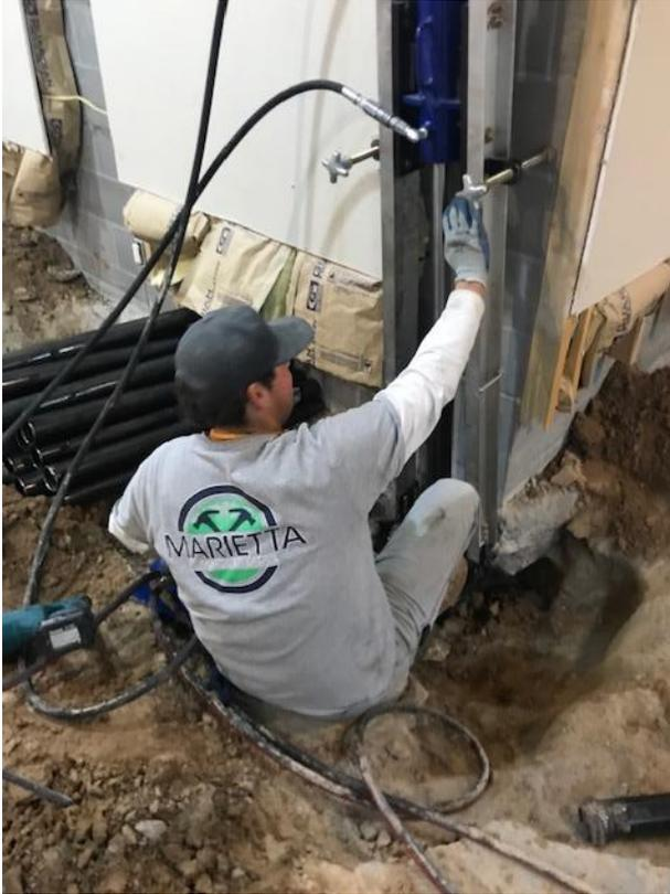
A total of 36 SafeBase Standard Duty Push Piers were installed with SaberTooth Brackets on the interior of the foundation to an average depth of 60' per pier. 170 linear feet of SafeBasements Waterproofing was also installed. The interior drain tile system consisted of SafeEdge Max and Multi-Flow drain tile with sump.
